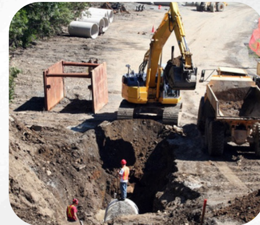
Pipeline Fabrication & Laying
